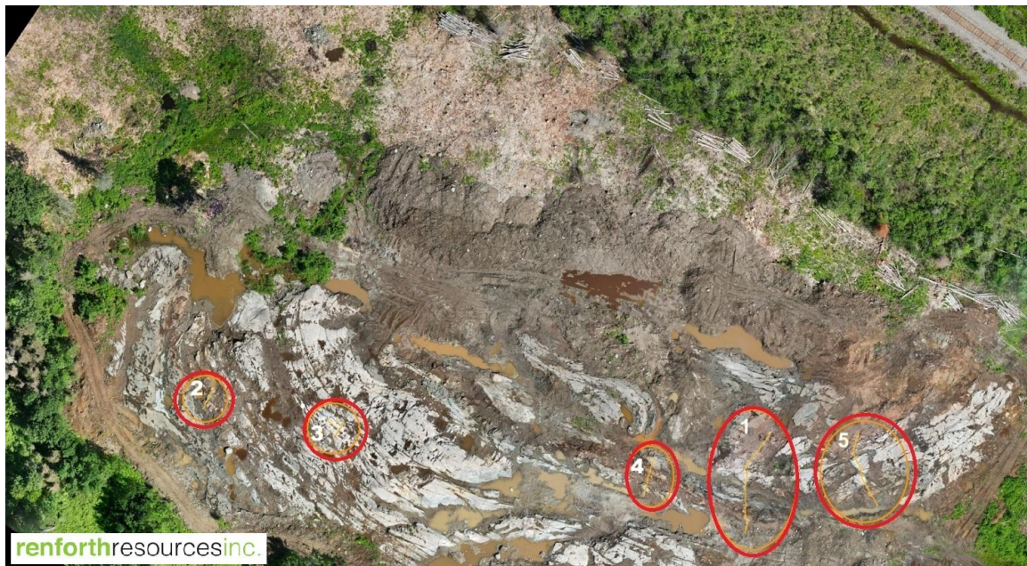
Detail of newly stripped area in Parbec's open pit footprint with channel areas 1 to 5 and trace of channels in orange
